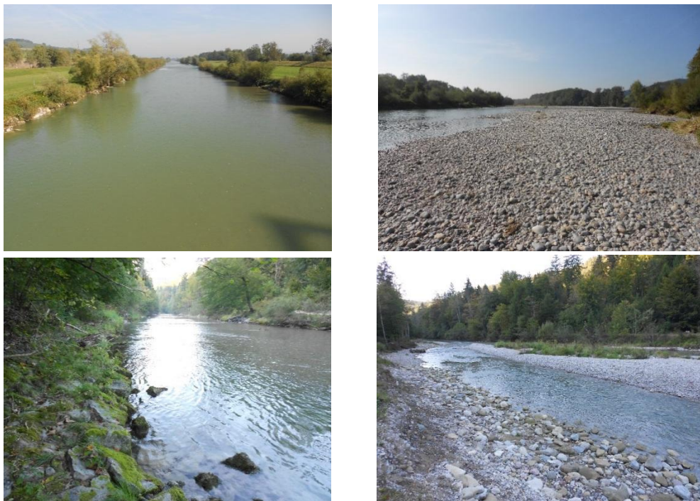
Figure 2. Illustration of channelized sections (left) and rehabilitated sections (right) of the Thur (top) and Töss (bottom) Rivers (pictures P. Reichert, Sept. 24, 2013; figure from Brouwer et al. 2015).
