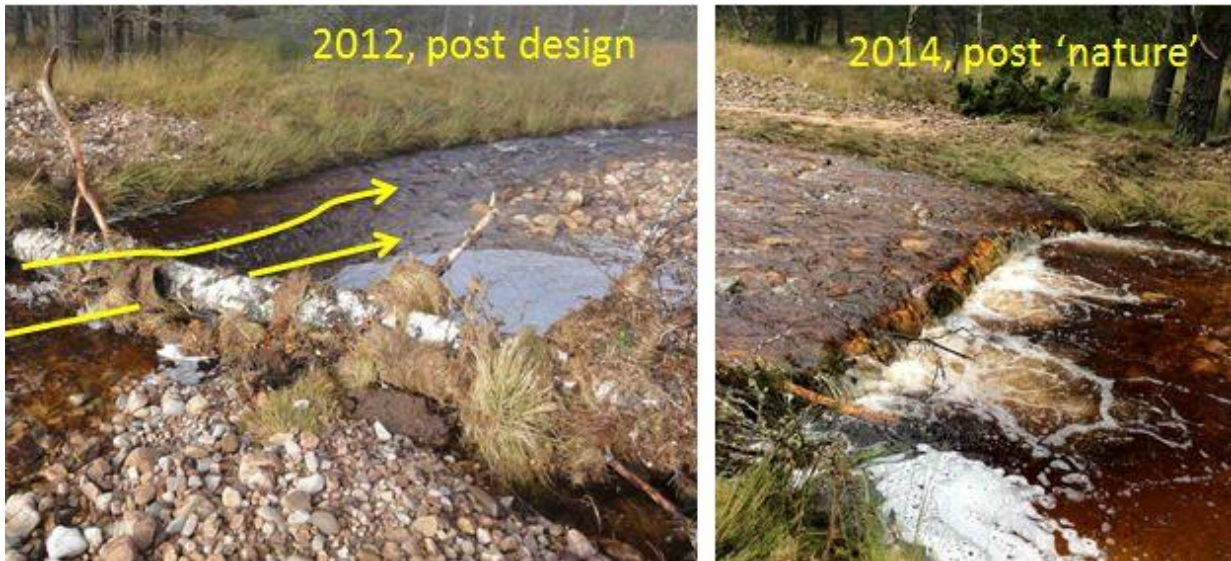
Figure 2. One of the large wood features introduced to the Allt Lorgy . Left: Channel spanning log showing complex post design flow paths, and large 3D perturbation to flow; Right: same log feature post-natural gravel transport; the wood feature is now more easily modelled in 2D.
