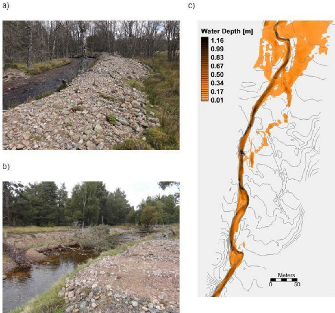
Figure 1. Improved floodplain reconnection predicted by model. Also shown is a relatively heterogeneous channel compared to a flume-like pre-restoration channel; a) image showing embankments found on pre-restoration reach; b) example of embankment removal and large wood placement; c) hydraulic inundation results showing floodplain connection. Flow is from bottom to top of figure.
