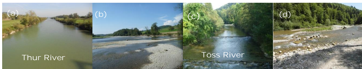
Figure 1. Illustration of channelized and restored sections of the Thur and Töss Rivers. Thur channelized (a), Thur restored (b), Töss channelized (c), Töss restored (d). Coordinates Thur: 47.5918 (N) 8.77114 (E) and Töss: 47.46338 (N) 8.72825 (E).
